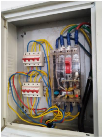
NC no inner cover installed
